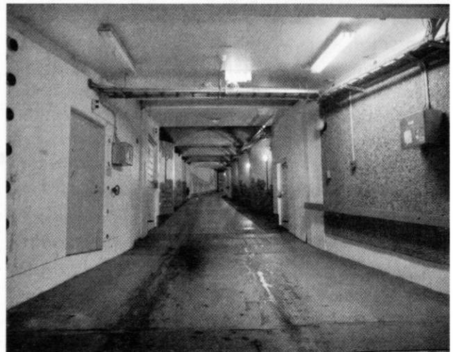
Vehicle entrance into the Mariaberget Civil Defence shelter in Stockholm.
